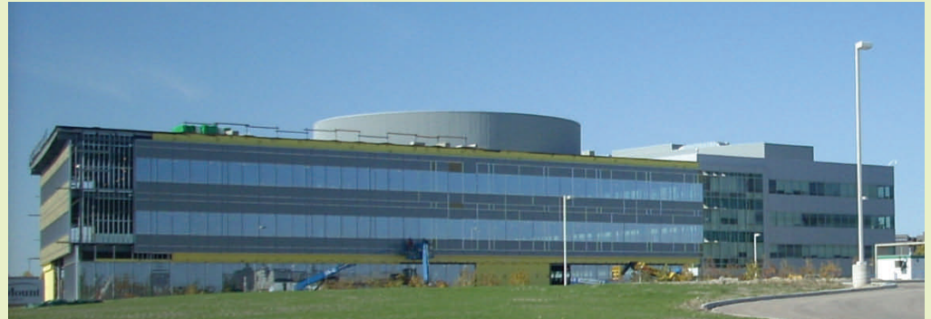
Westmount Corporate Campus ~ Carma Building Under Construction
