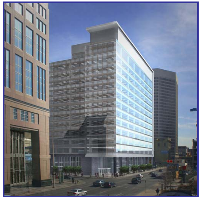
Artist's Rendering of Bankers Court, Calgary Co-owned by bcIMC and Brookfield Properties
